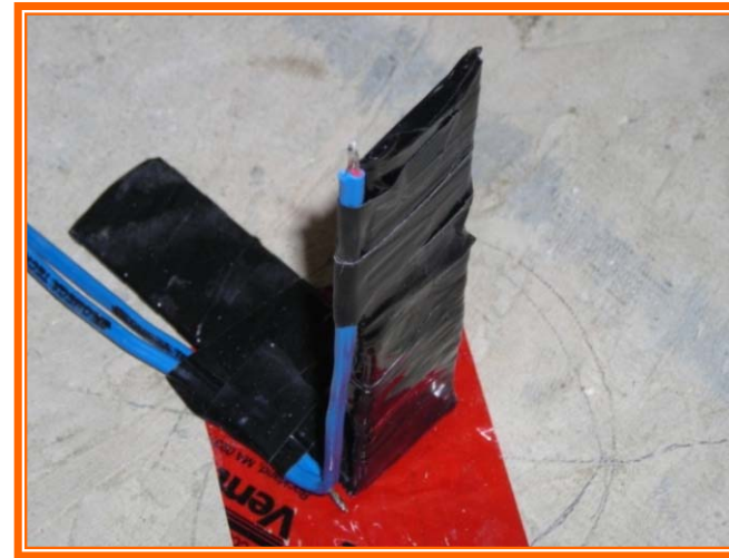
TC in the ground floor slab
