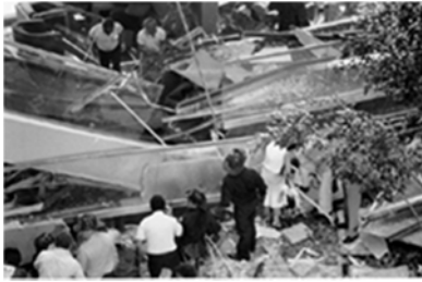
Overstressed steel support rods ( underdesigned )
