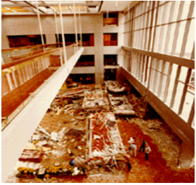
Hyatt Regency (KC) walkway collapse (1981)
