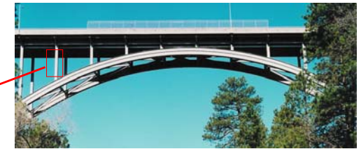
Canyon Bridge, Los Alamos, NM (photo courtesy P.M. Anderson)
