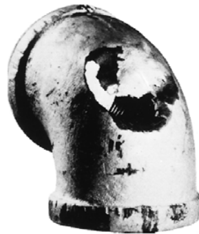
FIGURE 18.20 Impingement failure of an elbow that was part of a steam condensate line.
