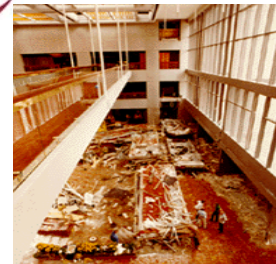
Hyatt Regency (KC) walkway collapse (1981)
