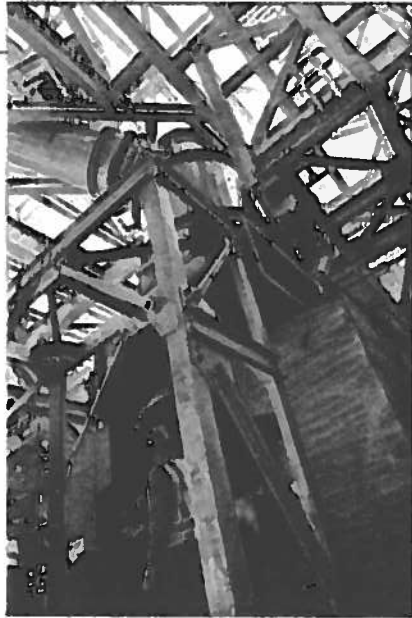
Gasifier at the 582 MW Kemper County plant.
