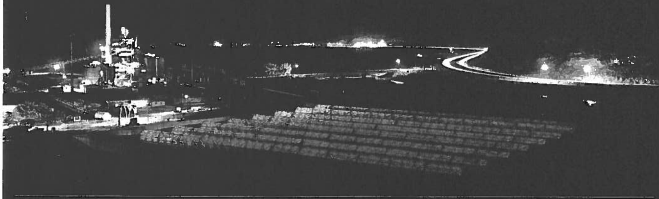
Xcel Energy's combined Cameo Station in southern Colorado ran a pilot program from July 2010 to Dec. 2010 that integrated concentrating solar generation until the Cameo plant was retired at the end of 2010. A parabolic trough solar field provided thermal energy to produce supplemental steam for power generation in order to decrease overall coal consumption, reduce emissions, improve plant efficiency, and test the commercial viability of concentrating solar integration. Courtesy: Xcel Energy
