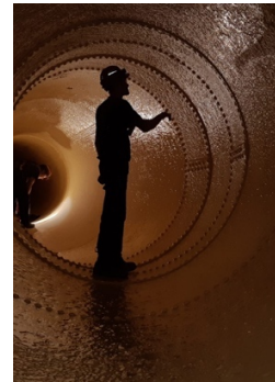
Figure 1.10. Hydroelectric dam and inside of the penstock. The evaluation of the pressure drop in the penstock is important to determine the power produced.
