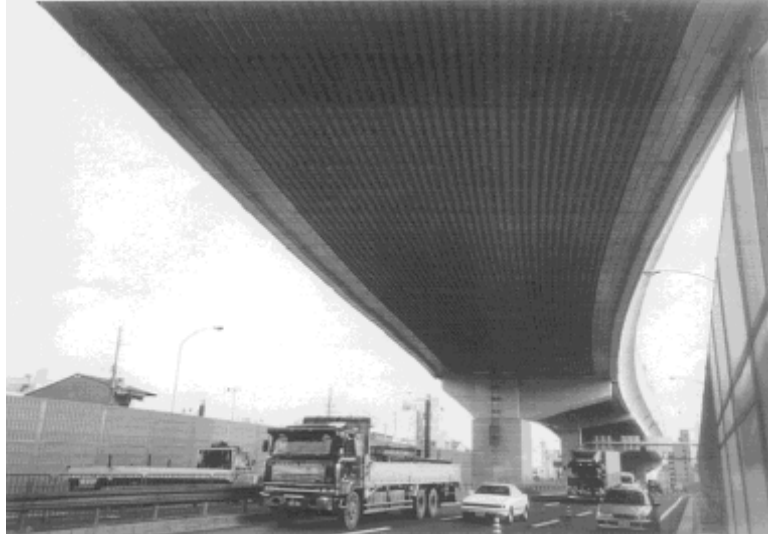
Figure 1.22: Sound absorbing structure on the under-side of an elevated viaduct [39].
