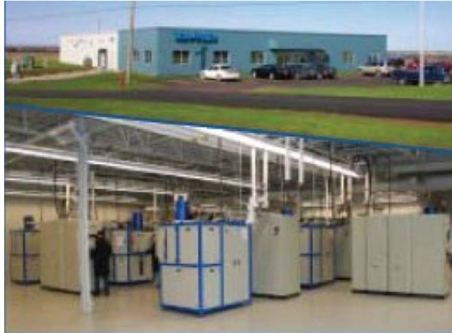
Figure 2-21 MDS-PRAD production facility in Prince Edward Island
