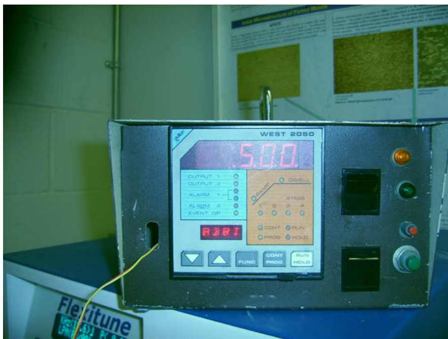
Figure 3-13: Digital temperature monitor.
